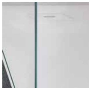
Glued glass-glass connection (not mitred)
