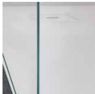
○ Glued glass-glass connection (not mitred)
