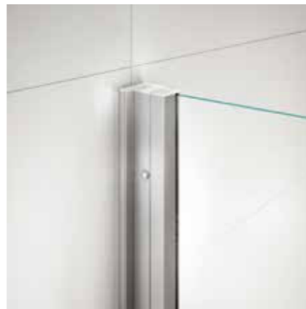
Interior view of the wall profile
